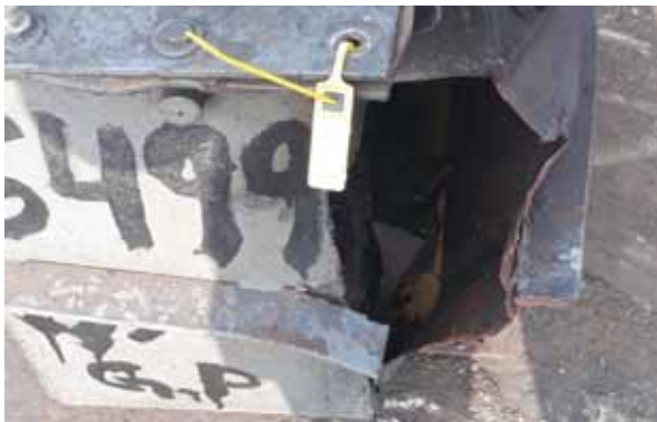
Opening of welding joint from one of the edges breaking stiffener also
