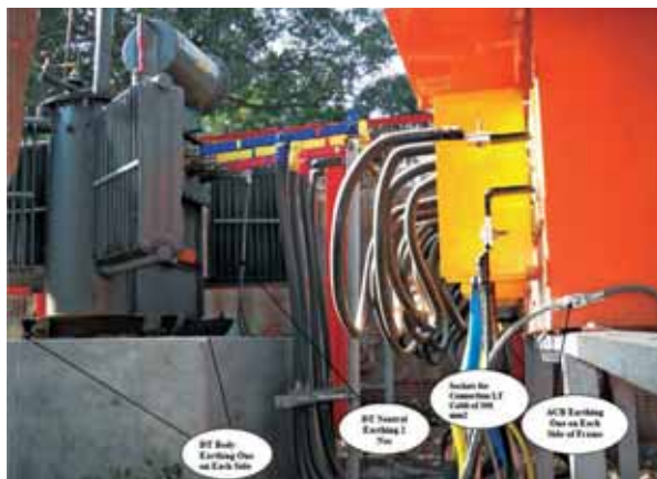
Fig 3: earthing of distribution transformer
