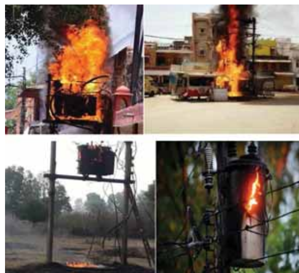
Fig 4: distribution transformers on fire
